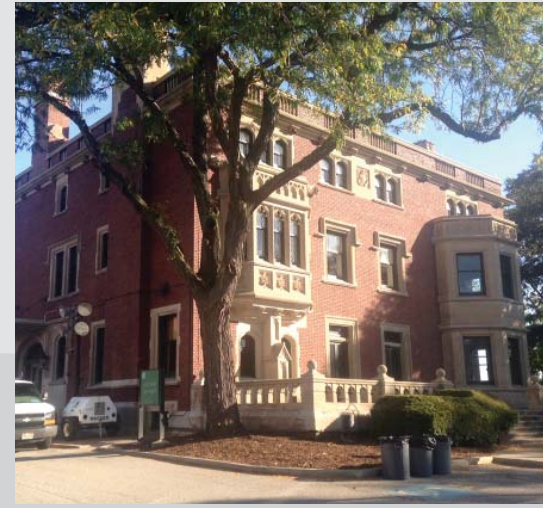
Mather Mansion Renovations Cleveland State University (After)
