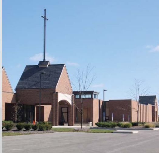
Church of the Beloved Disciple Grove City, Pennsylvania
