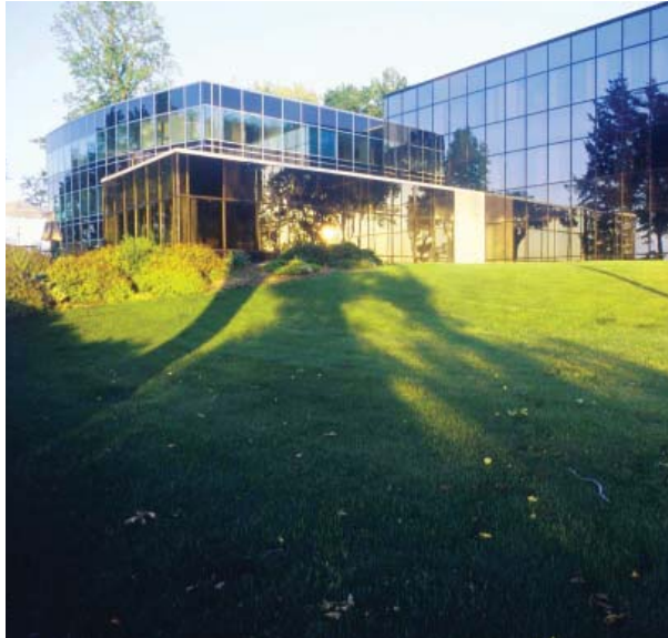
Rentway Corporate Office Addition Erie, Pennsylvania
