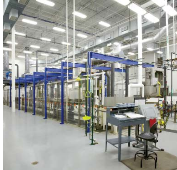
LORD Corporation Robison Road Facility Erie, Pennsylvania
